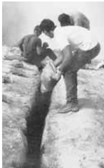
Figure 23. GEM permanent ground enhancement material, is ideal in areas of poor conductivity and is suitable for both backfilling around ground rods and trench installations.
